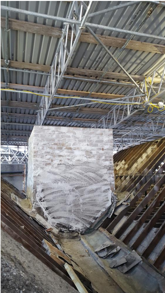
Repaired chimneybreast before application of render (Photo: J. Donnelly)
