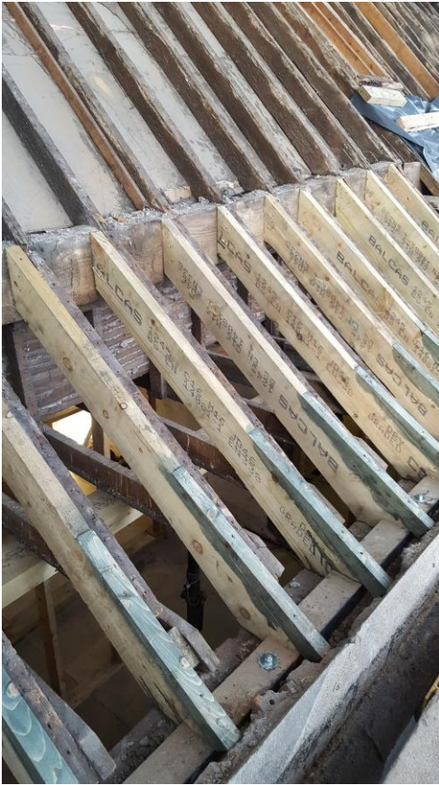
Companion rafters in place (Photo: J. Donnelly)
