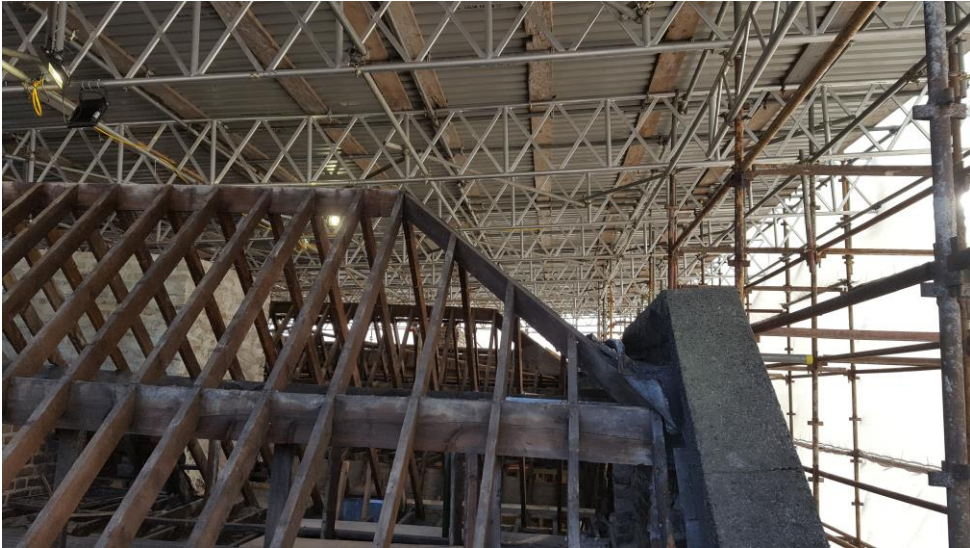
Rafters exposed with over-roof in place (Photo: J. Donnelly)
