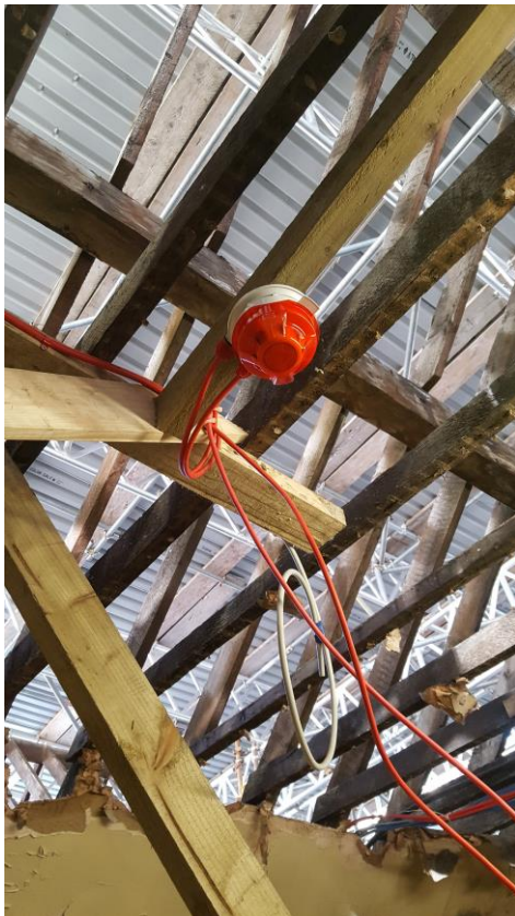
Fixing of temporary electrics (Photo: J. Donnelly)
